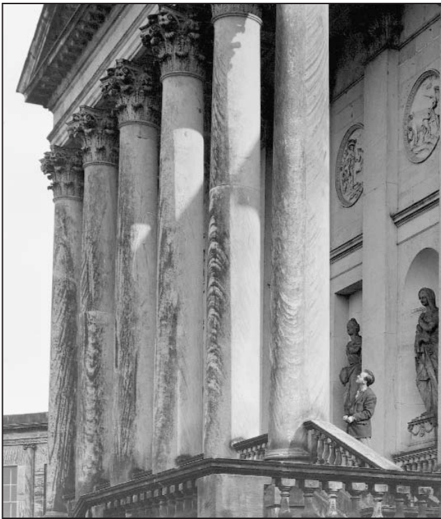
Figure 3. Kedleston Hall, Derbyshire, built 1759-63: north portico with massive columns of cross-bedded sandstone quarried from the Crawshaw Sandstone at Horseley Castle (BGS photo #L892, 1966).
